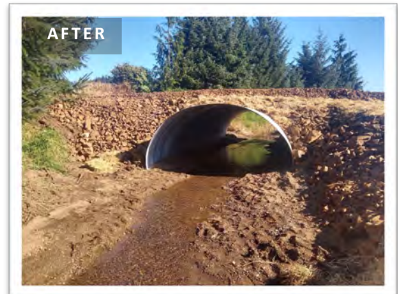
AFTER: One of three new arch culverts.
