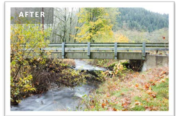
AFTER: The new 32' bridge allows unimpeded fish passage, and ample capacity to pass high flows and debris during storm events.
