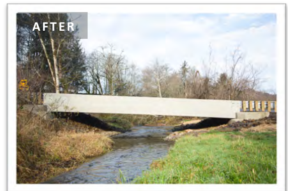
AFTER: The new 52' bridge allows unimpeded fish passage, and ample capacity to pass high flows and debris during storm events.
