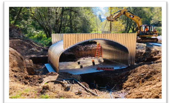
DURING: The prefabricated aluminum box culvert was assembled on site.
