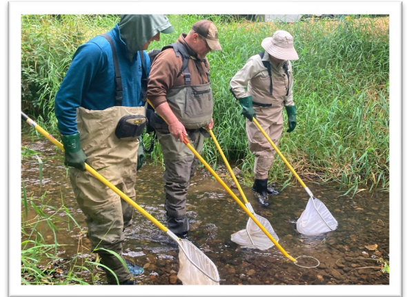
BEFORE: Aquatic organisms were relocated from the project area prior to construction.
